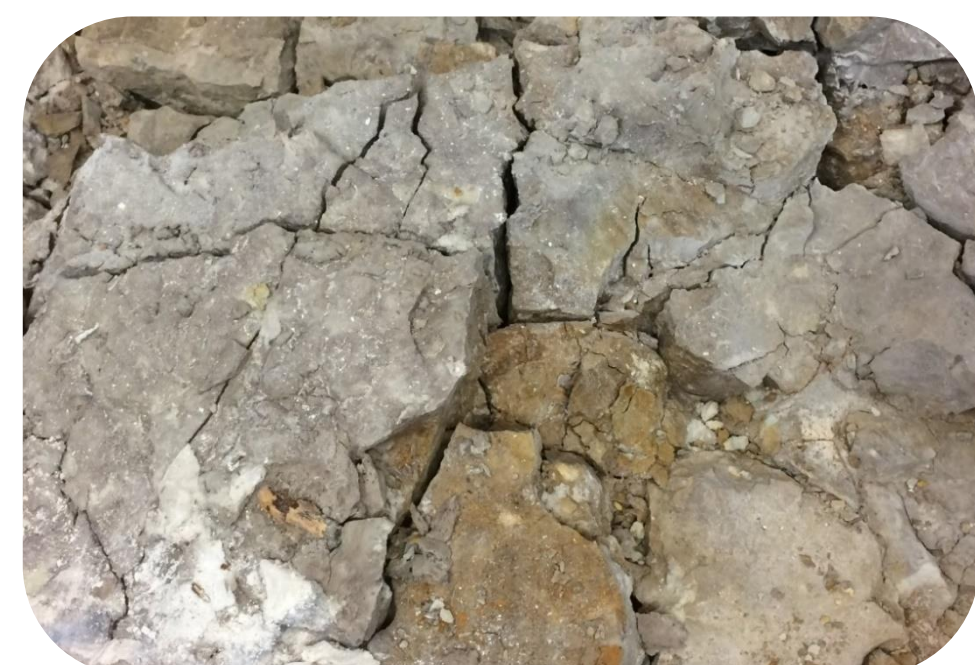
Multiple desiccation cracks form if the site is exposed for a prolonged period, negatively affecting the fossils.
