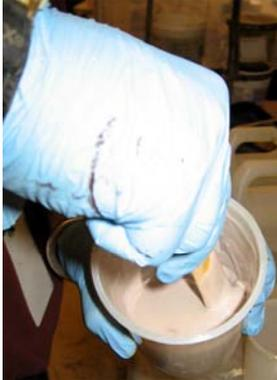
**Stir together the resin and colour until thoroughly mixed. Remember, the more mixing you do, the more air you add to the epoxy mixture.**
