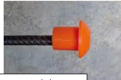
Safety caps are recommended over the end of the rebar to protect against impalement!
